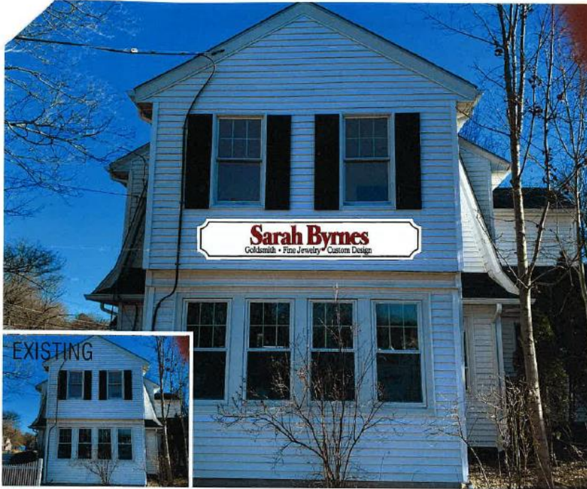
Existing Wall Sign (west side of building)
