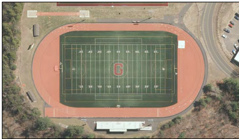
Existing Conditions Aerial
