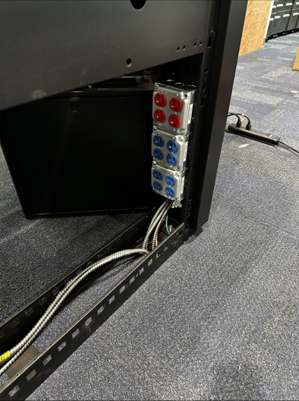
1 JUNCTION BOX BKT MOUNTS TO THE END OF THE FLEX WALL FRAME. VERTICAL SPACE FOR UP TO 3 JUNCTION BOXES AS SHOWN.
