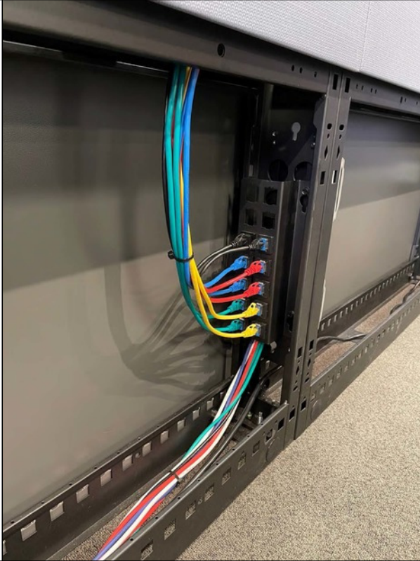
2 DATA TERMINATION BKT MOUNTS VERTICALLY TO THE END OF ANY FLEX WALL. HAS SPACE FOR UP TO 14 KEYSTONES.
