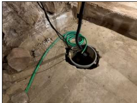
Sump pump on eastern side of basement
